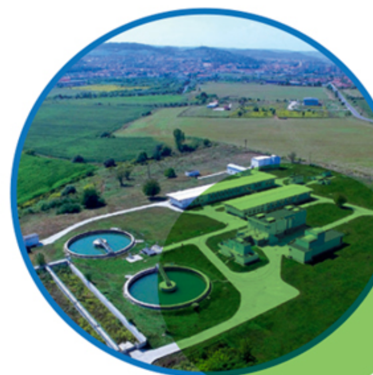
Drinking water treatment plant
